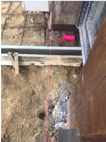
303 N. Washington Avenue, today's site preparation to pour over the property line without a break at the property line. (Additionally, the footer was covered with dirt.)
