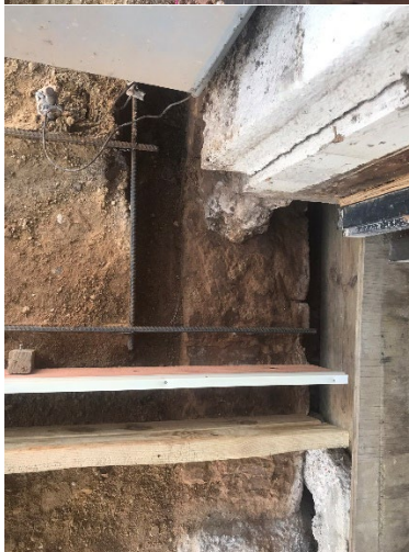
303 N. Washington Avenue uncovered existing footer which directly lines up with the neighboring storefronts.
